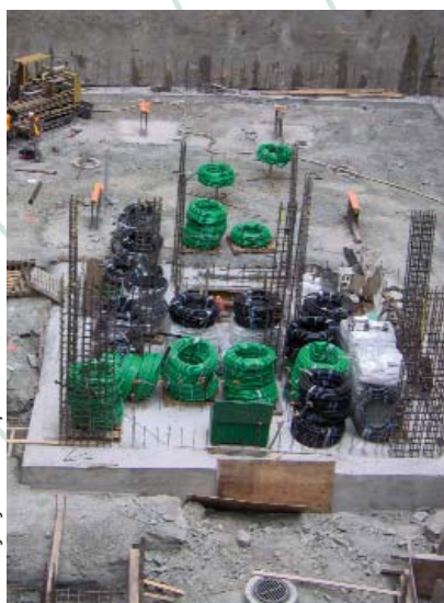
A drilling project for a vertical borehole ground heat exchanger for a mixed use residential/retail building
