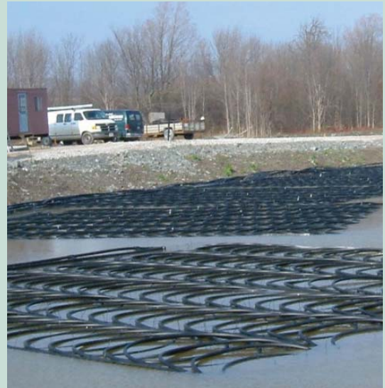
Installation of a closed lake loop for a commercial application
